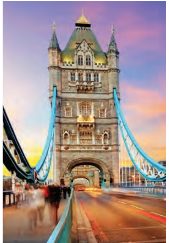
Step inside London's Tower Bridge and see the Victorian Engine Rooms.
